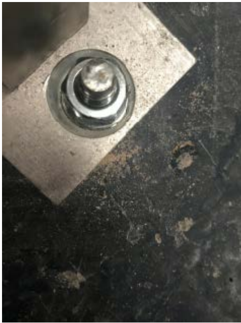
Figure 1a: M10 Projecting Bolt Anchors with M10 washer and M10 nut.
